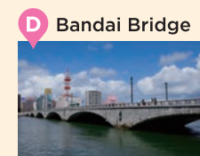
D Bandai Bridge A symbol of Niigata City, also designated as an Important Cultural Property.
